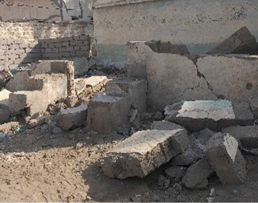
One of the homes before being rehabilitated
